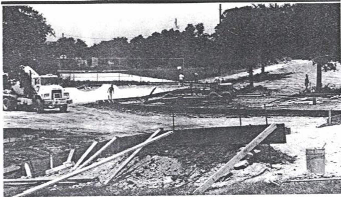
Construction should be completed at the RW pool within 30 days. Photo by Bonnie S. George
